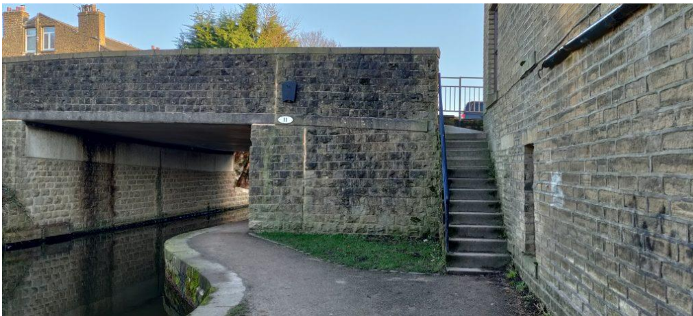
Steps by bridge no. 11
